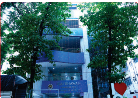
Lighting to Building
